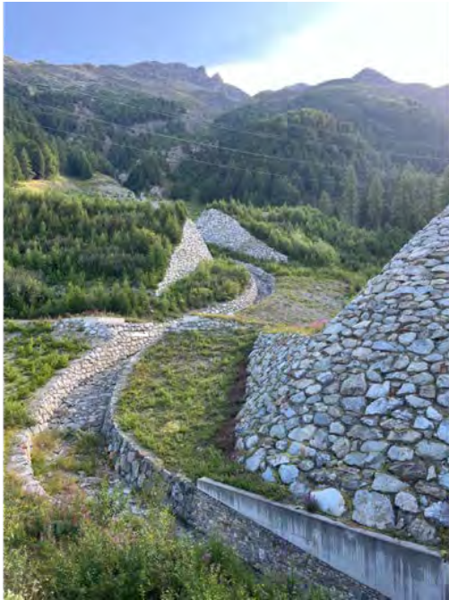
Figure 1: Auffangdämme of Pontresina, Switzerland
