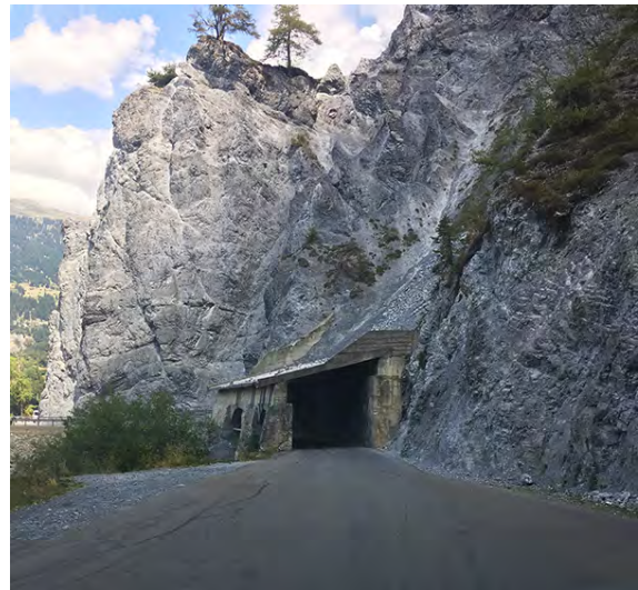
Fig.8 Tunnel built into cliff to protect against sliding rocks
